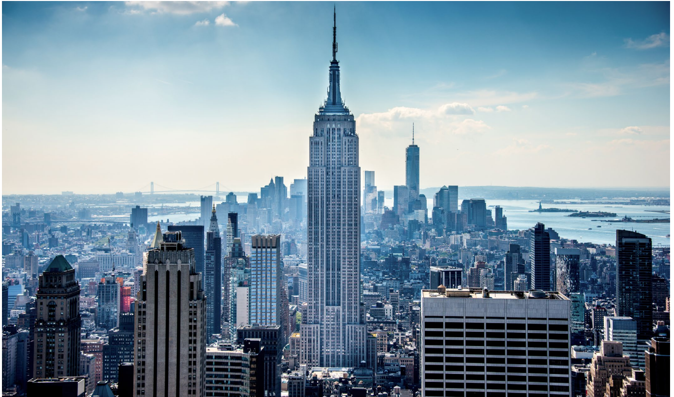
$800,000 annual energy savings at the Empire State Building
