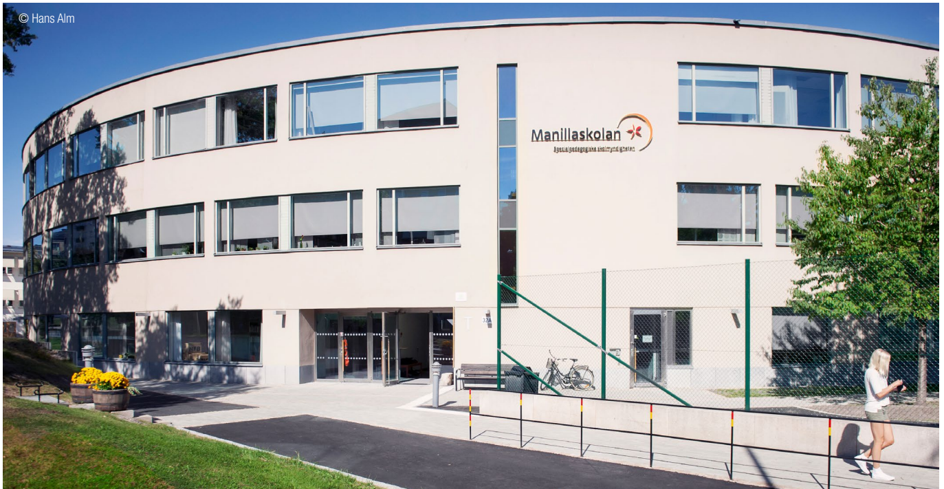
Die Wireless-BACnet-Technologie reduzierte die Installationszeit um 65 %. Wireless BACnet technology reduced the installation time with 65%.
